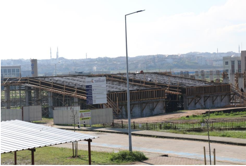
green roof (Gebze Technical University)
